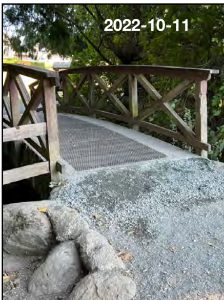
Repaired bridge ramp
